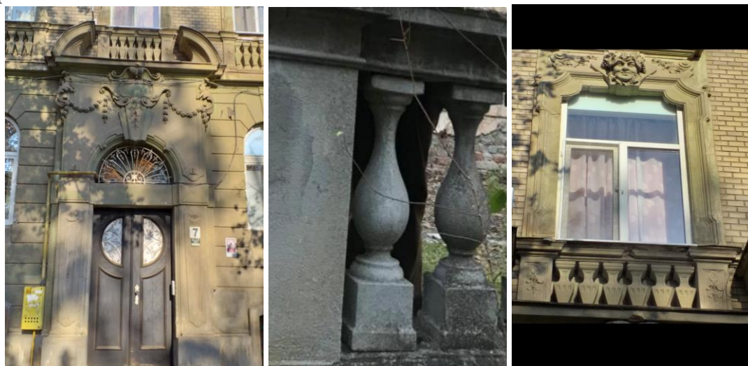
Figure 5 Pilasters at buildings from 3 August 1919 street
